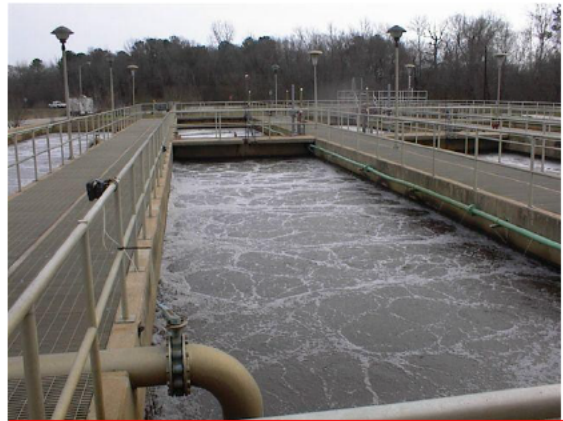
Wastewater Treatment Plant Aeration Basin
