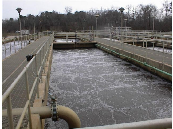
Wastewater Treatment Plant Aeration Basin
