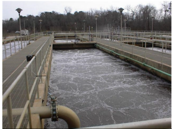
Wastewater Treatment Plant Aeration Basin
