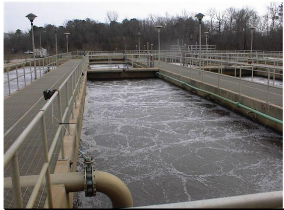
Wastewater Treatment Plant Aeration Basin
