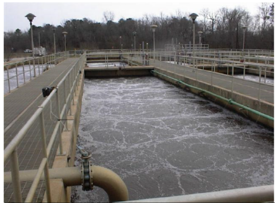
Wastewater Treatment Plant Aeration Basin
