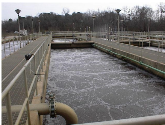
Wastewater Treatment Plant Aeration Basin
