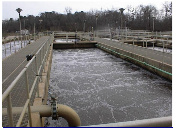
Wastewater Treatment Plant Aeration Basin
