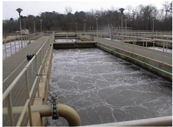
Wastewater Treatment Plant Aeration Basin
