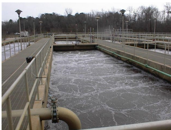
Wastewater Treatment Plant Aeration Basin
