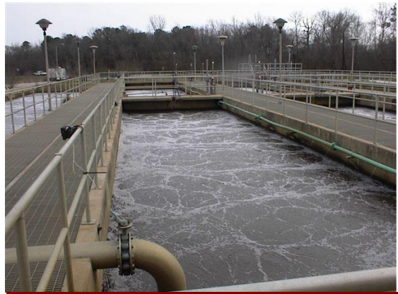
Wastewater Treatment Plant Aeration Basin
