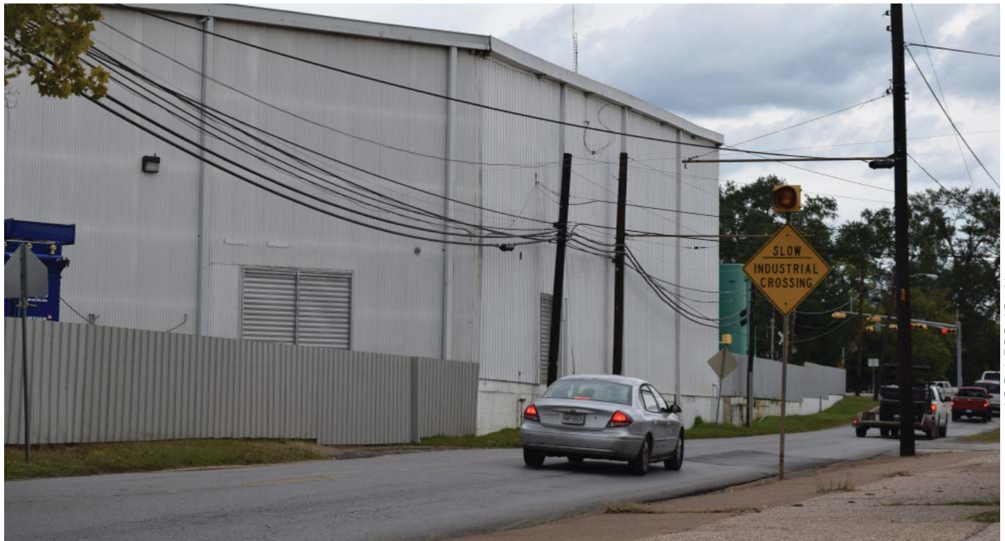
Lufkin Industries brownfield site opportunities to redevelop a mixed use, public/private development
