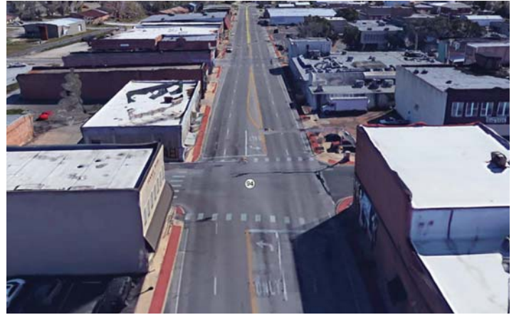
Existing Frank Avenue Downtown Streetscape from 1st Street to 4th Street.
