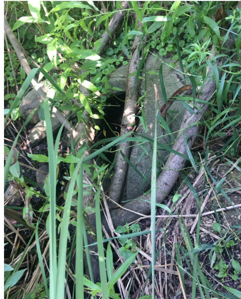
Willow Drain (W22-00) (Franklin Farms Phase 2) Photo Date: 20190722 View of the 12-inch storm drain inlet in the detention basin identified as Inlet L-2 on Sheet C5 of the Wolverine plans. Inlet is overgrown and nearly plugged with vegetation.
