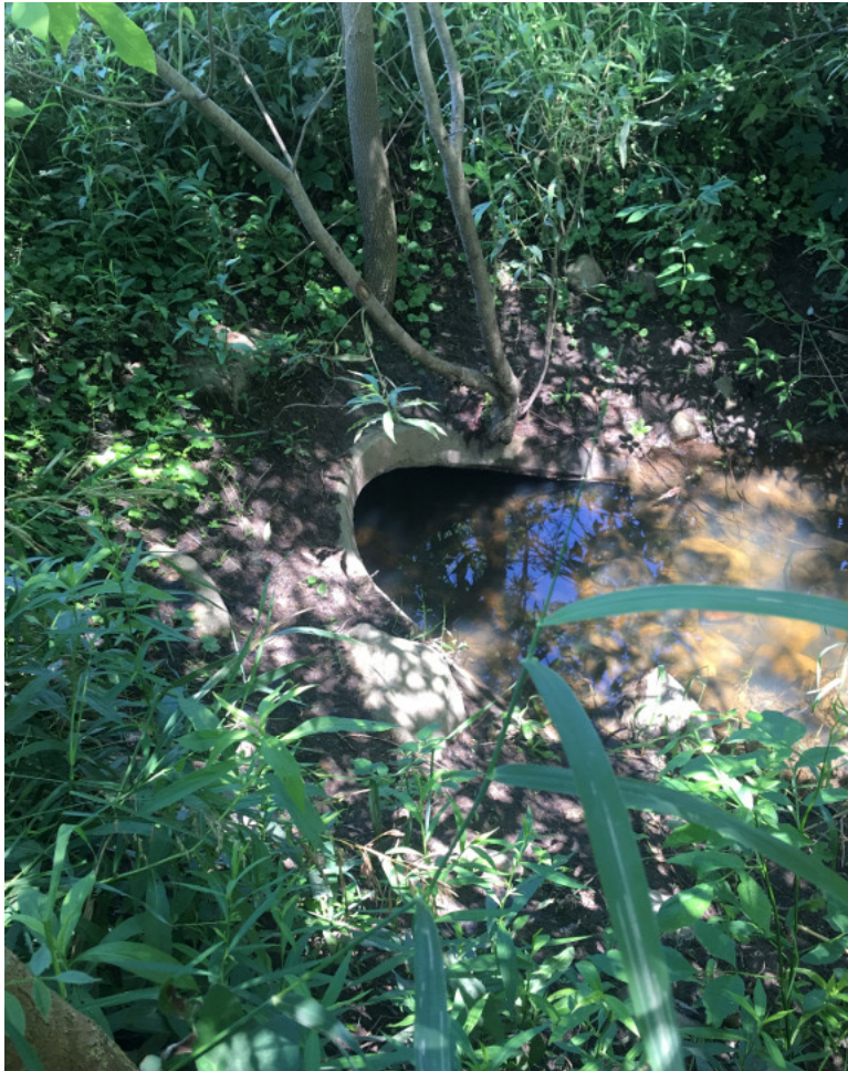
Willow Drain (W22-00) (Franklin Farms Phase 2) Photo Date: 20190722 View of the 18-inch storm drain outlet identified as Outlet L-3 on Sheet C4 of the Wolverine plans. Outlet is open but partially plugged with sediment.
