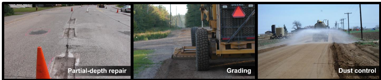
Figure 6: Examples of capital preventive maintenance treatments, cont'd—(from left) concrete road prepared for partial-depth repair, gravel road undergoing maintenance grading, and gravel road receiving dust control application (dust control photo courtesy of Weld County, Colorado, weldgov.com).
