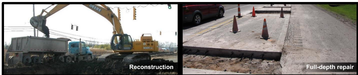
Figure 3: Examples of reconstruction treatments—(left) reconstructing a road and (right) road prepared for full-depth repair.
