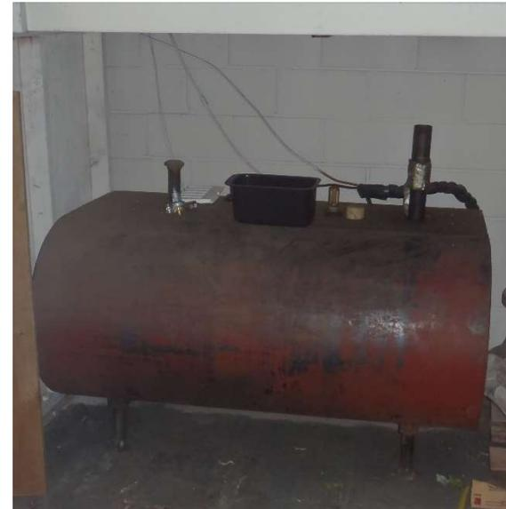
Figure 49: Above Ground Storage Tank (Source: T&M)
