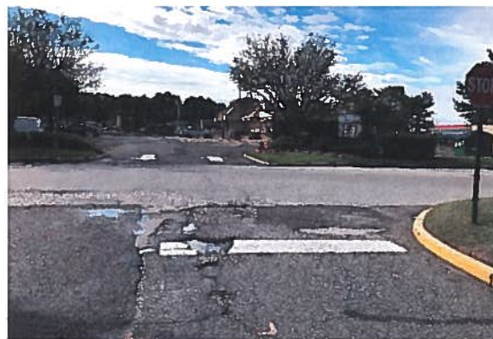
Deteriorating pavement conditions within the ShopRite Shopping Center (Block 302.15, Lot 12)
