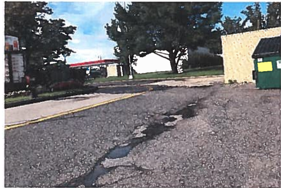
Pavement conditions and exposed trash enclosure on Lot 12.03 (McDonald's)
