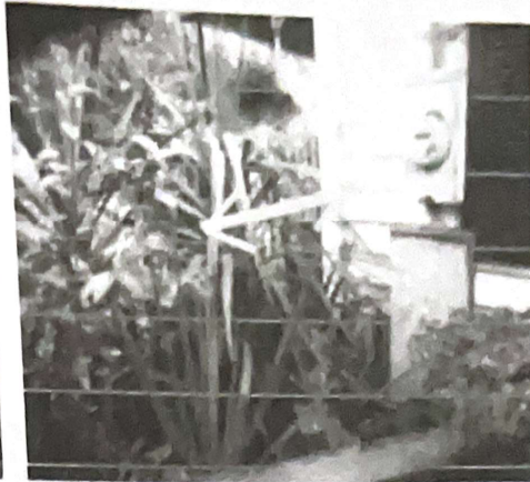
Photo 5-2 Remove ALL plantings away from the structure 4-5 feet to prevent insect infestation, and moss or mold growth.
