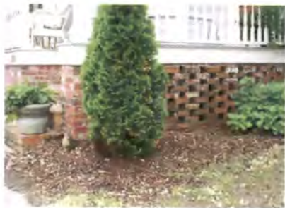
An example of brick lattice
