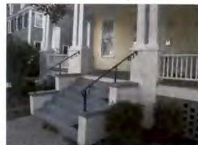
The metal stair railing was added to this porch stair as a safety feature. The use of a simple metal design does not detract from the historic porch and identifies it as a later addition.
