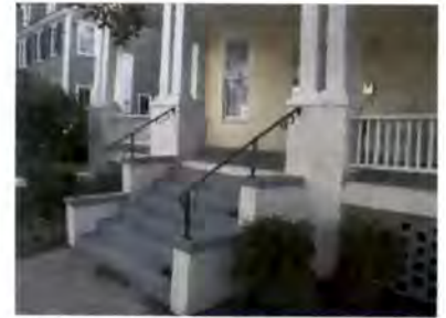
The metal stair railing was added to this porch stair as a safety feature. The use of a simple metal design does not detract from the historic porch and identifies it as a later addition
