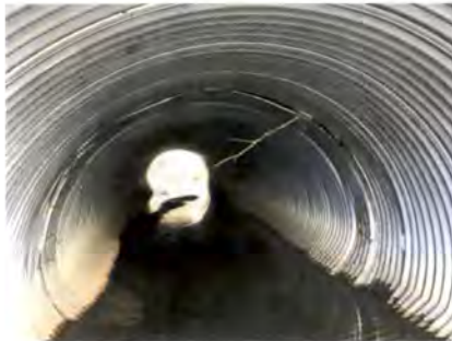
JOINT REPAIR INSIDE 36"X72" ALUMINUM BOX CULVERT
