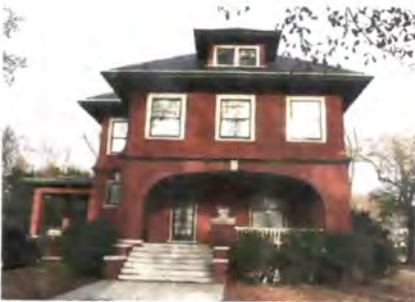
This house in the Riverside Historic District has a brick masonry veneer at the first floor and wood shingle siding at the second floor.
