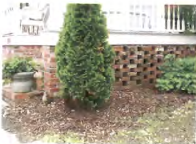
An example of brick lattice.
