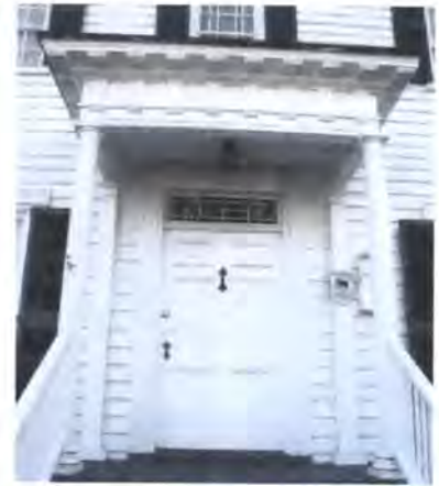
The door, transom, molded surround, corner blocks, pilasters, columns, entablature, flat roof, and stair combine to compose this fine entrance.
