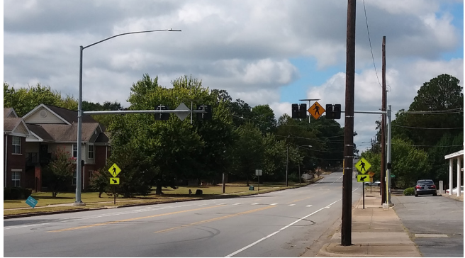
Pedestrian Hybrid Beacons stop automobile traffic for bicyclists and pedestrians wishing to cross a high traffic volume/high speed roadway.
