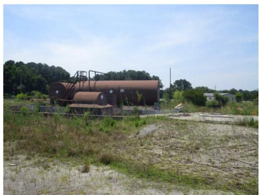
Photo 10 A view of two large ASTs near the central portion of the site confined within a concrete containment structure.
