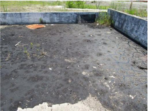
Photo 14 A view of black staining and residue within the concrete containment structure that confined the ASTs labeled Off-Road Diesel near the central portion of the site.
