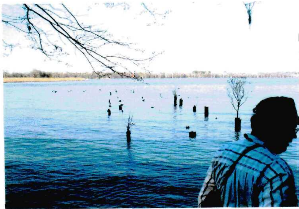
Camp Battle - Piers for dock at shoreline of the Neuse River. NOTE: planks are completely gone and southeast end of Marsh Island in left background.
