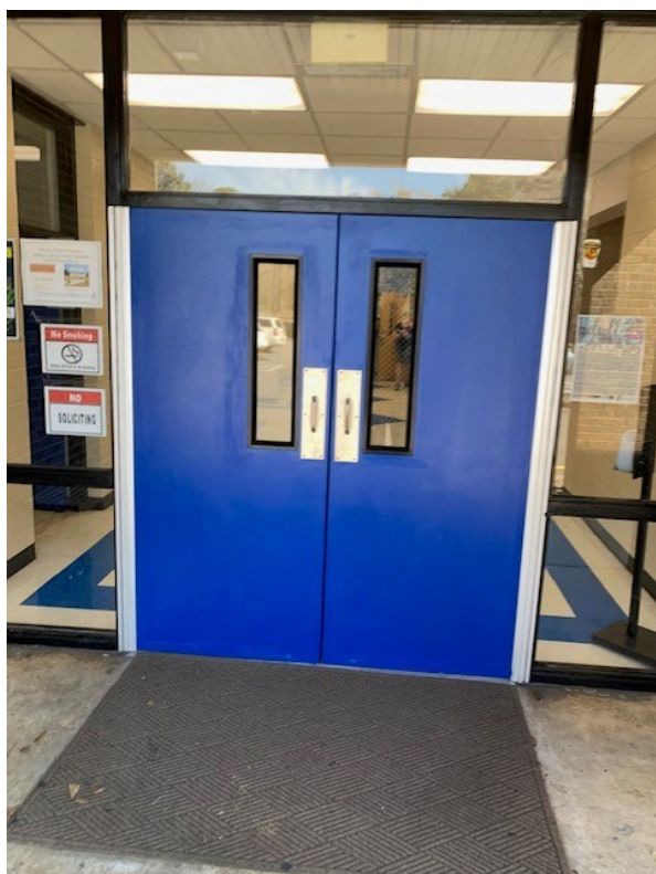
Mat at entrance is not securely attached on the edges.
