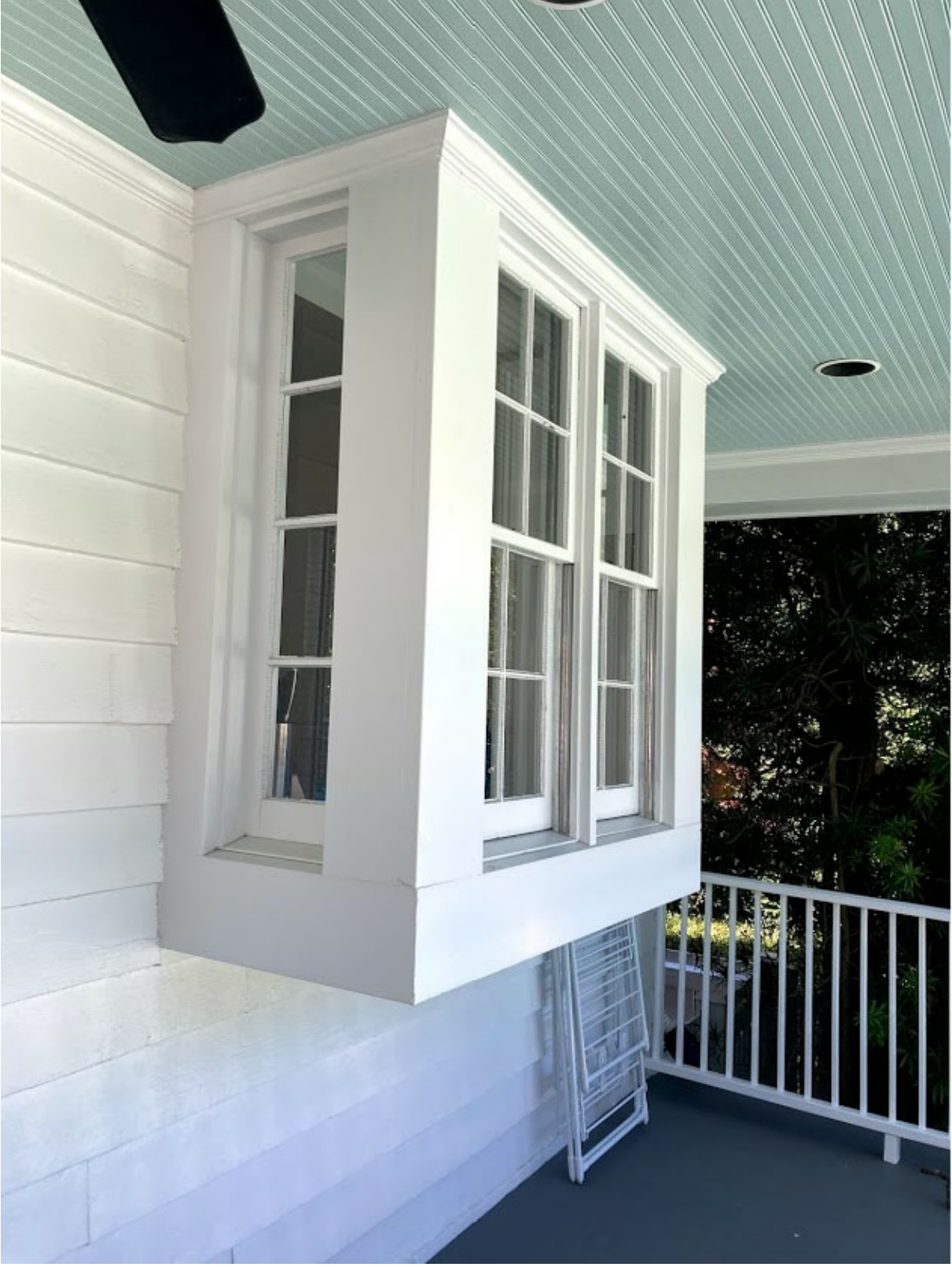
PHOTO 9 - DEMO WINDOW BOX AND INSTALL NEW 1 OVER 1 WOOD WINDOW
