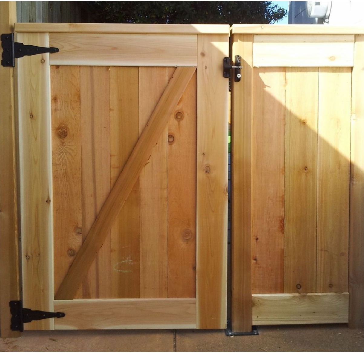
EXAMPLE OF WOOD PRIVACY GATE. NEW GATE TO HAVE (2) 4' X 6' PANELS PAINTED WHITE
