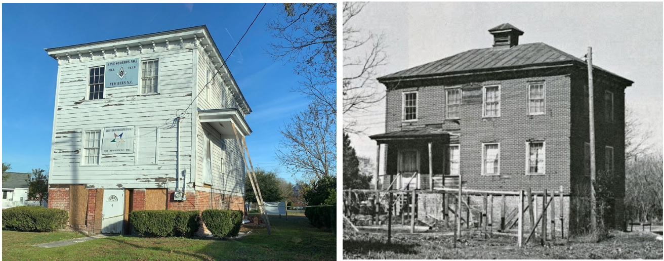
Figure 6.4. King Solomon's Lodge, taken during site visit December 2020
