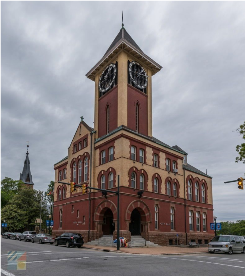
Figure 6.2. New Bern Municipal Building
