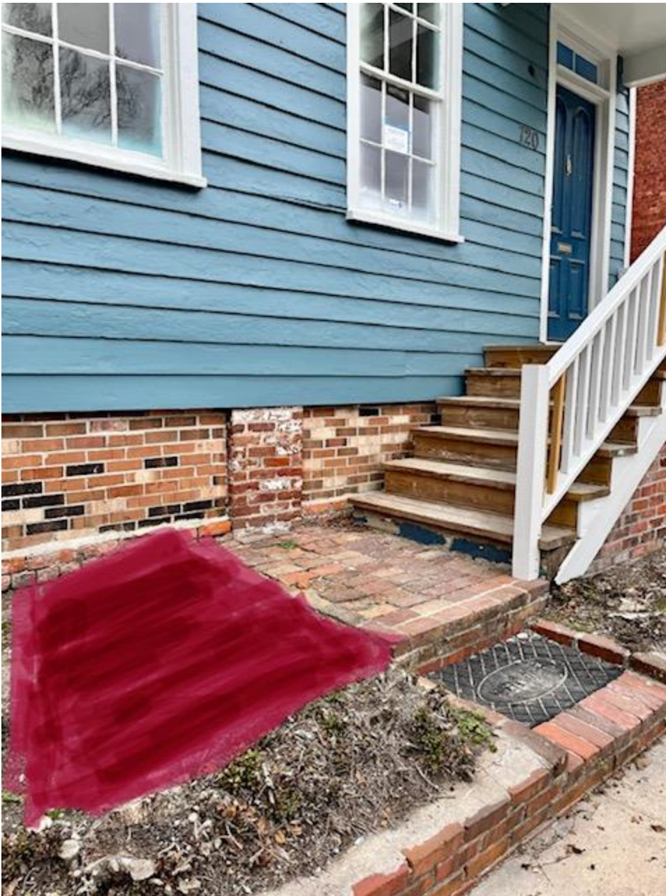
The area marked in red will be brick – there is some brick in this area as this appeared to be brick at some time. We will reuse what we can and match the rest.
