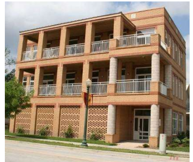
This building is located in the transitional edge between dense fabric and tight weave development patterns. The use of a modern blonde brick and patterned masonry is appropriate for this infill construction.
