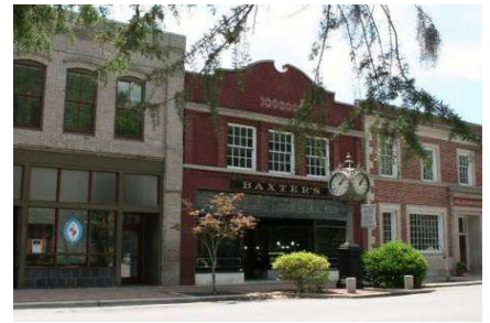
Baxter's unique curved coping creates visual interest when compared to the parapets and cornice lines of surrounding buildings.
