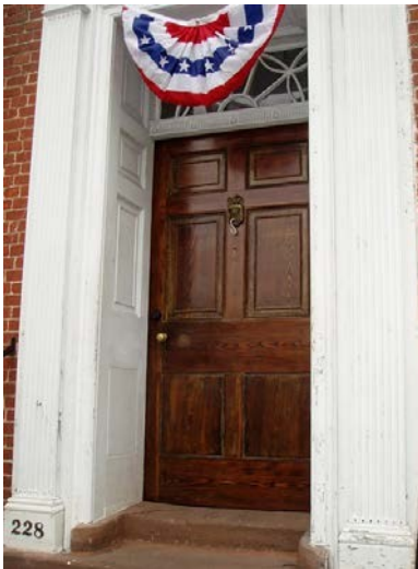
An example of a historic wood door that has been appropriately repaired instead of replaced.
