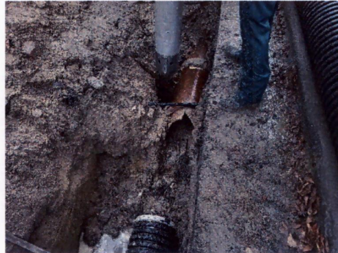
Collapsed Pipe on Middle Street
