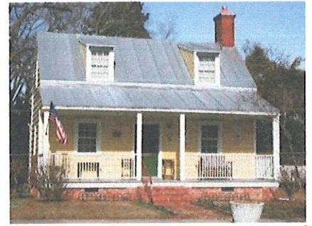
Standing seam metal is a common roof material in the historic districts resulting from reduced insurance rates following the Great Fire of 1922.
