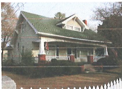
The brick piers and tapered posts are characteristic of the Craftsman Bungalow style of architecture.
