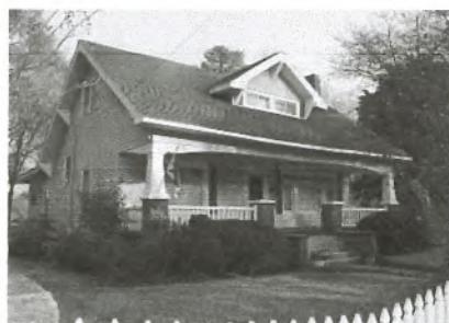
The brick piers and tapered posts are characteristic of the Craftsman Bungalow style of architecture.
