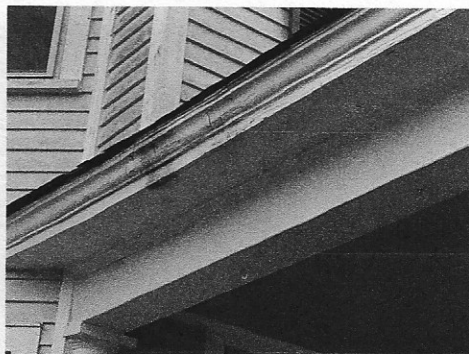
Picture #4: current leak and rot on roof
