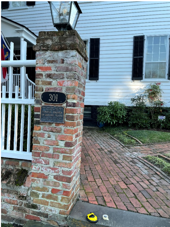
Front entry off Johnson Street, Entry columns are spaced 52" apart and 69" to bottom of crown, 77" to top
