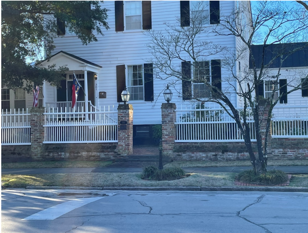
Front entry off Johnson Street, Entry columns are spaced 52" apart and 69" to bottom of crown, 77" to top
