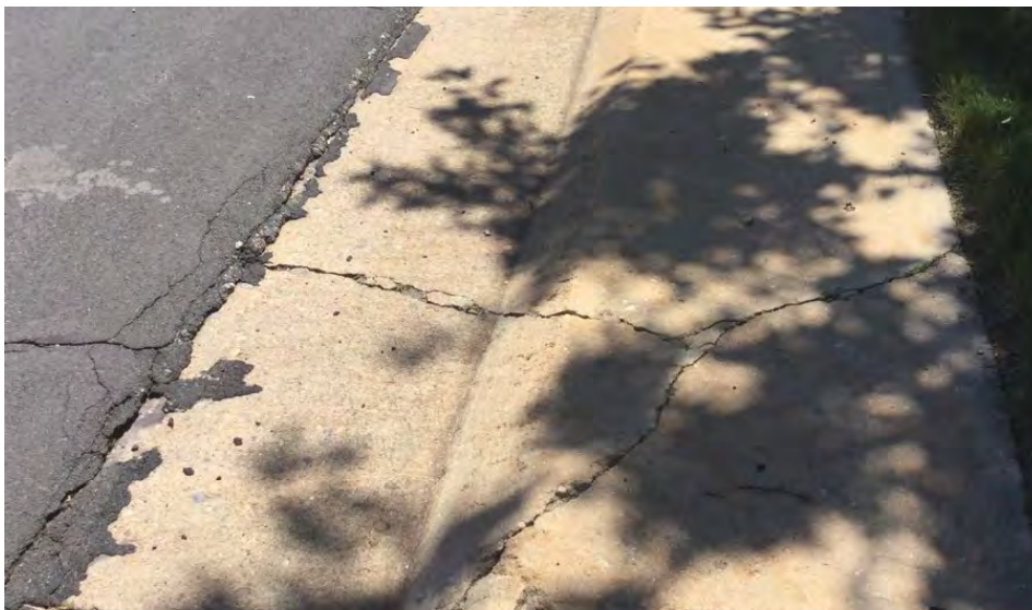
Section of sidewalk and gutter showing need for replacement
