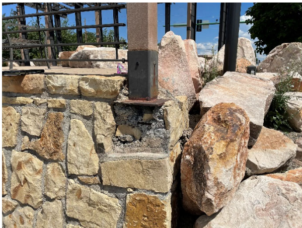
Retaining Wall Stone Repair (Bid Alternate Item 18)
