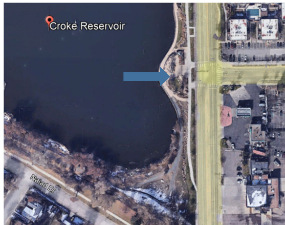
Location of Retaining Wall Stone Repair (Bid Alternate Item 18)
