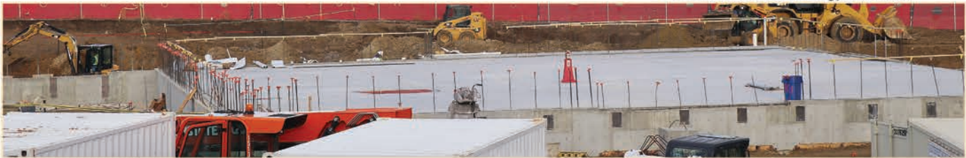
▼ Concrete slab for the gymnasium
