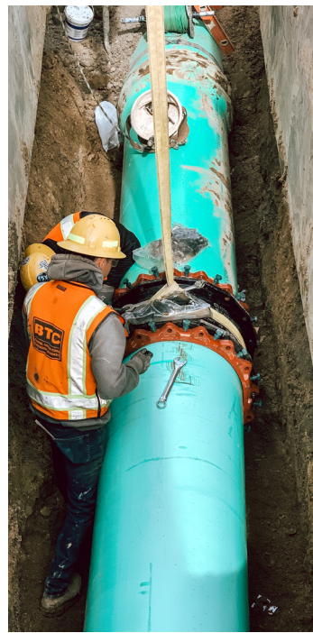
BT Construction crew members work on a tie-in of the pipes on the Force Main A project.
