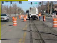
Construction Crews Working on Huron Street
