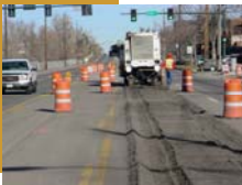
Construction Crews Working on Huron Street
