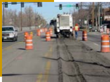
Construction Crews Working on Huron Street
