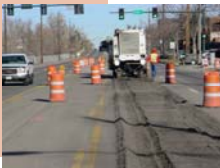
Construction Crews Working on Huron Street
