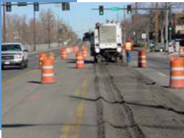
Construction Crews Working on Huron Street
