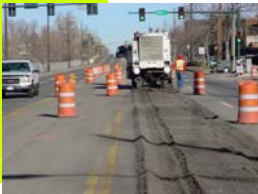
Construction Crews Working on Huron Street
