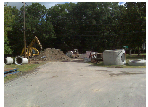
Construction of new Sewer
