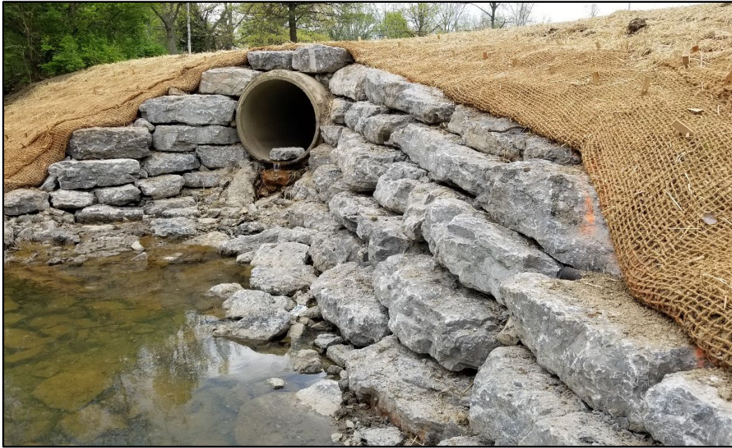
Photo 4 Example of imbricated riprap outfall protection constructed in Brooklyn, Ohio.
