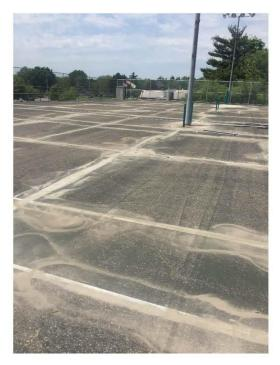
The asphalt surface was then prepped, filled and leveled in preparation for a new topcoat
