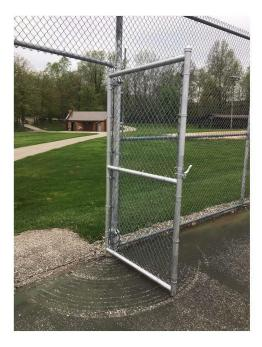
17,535.00 Of fence repairs were done including new bottom and mid rails and repair and restting of all the gates.
