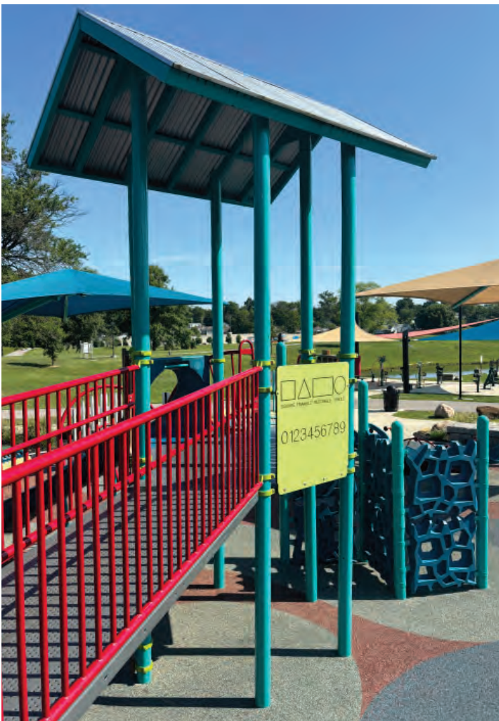
Tripton Park was designed with accessibility in mind. Image Source: HWC Engineering
