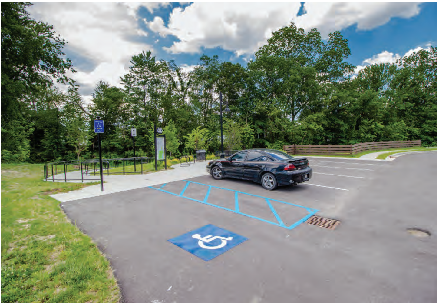
A ramp at the Muscatatuck Trailhead connects the paved trail to an accessible parking space. Image Source: HWC Engineering
