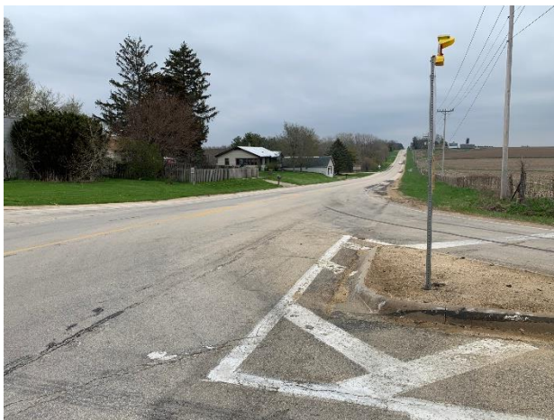
Lowell Park Road Northbound Looking East – >1,200'
