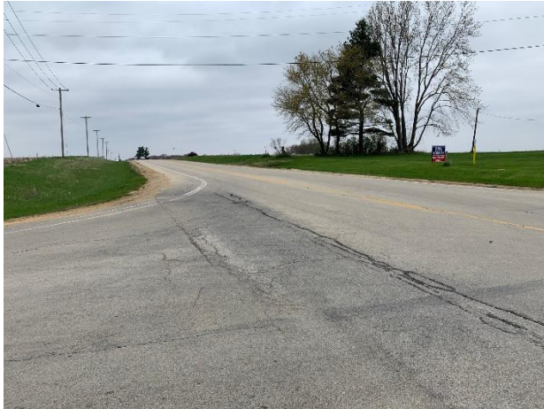
Lowell Park Rd Northbound Looking West – 750’
