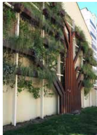
Vertical Tree Garden, Urbanarbolismo
