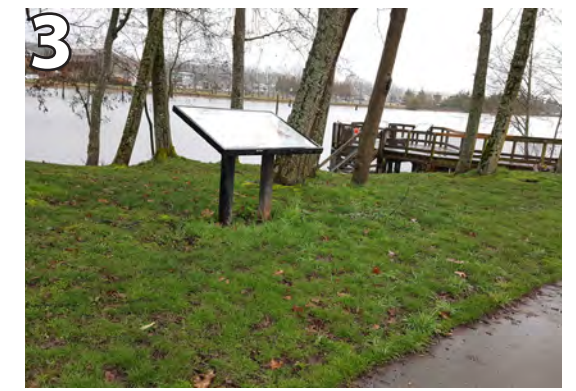
Interpretive signage not accessible. Relocate next to sidewalk or provide ADA accessible pathway.
