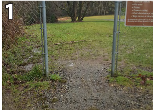
No ADA accessible parking space. Provide ADA accessible parking space
