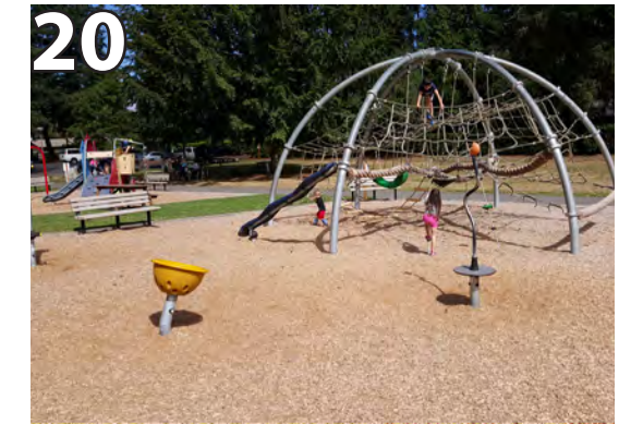
20 EWF is very worn down in both play areas. Especially around the play equipment making the spaces non-ADA complaint.
