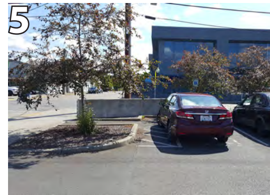
5 Inadequate ADA parking. Provide (3) ADA accessible parking spaces. (1) must be van accessible and have proper signage.
