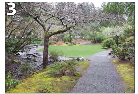
Cross slope near trail intersection is 3.5%. Regrade so cross slope is less than 2.08%.
