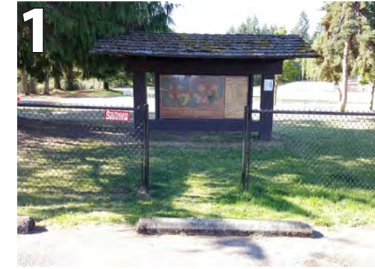
Kiosk not accessible from parking lot. Provide ADA compliant pathway.
