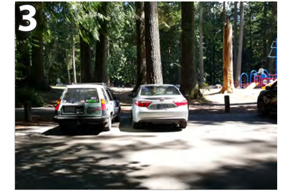
3 No ADA parking space for shelter #4. Re-strip to provide for (1) accessible space. Install signage
