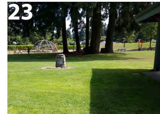
23 Drinking fountain not accessible. Replace with compliant drinking fountain and provide ADA pathway.
