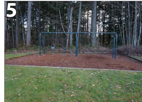
5 Provide ADA compliant pathway to swing sets.
