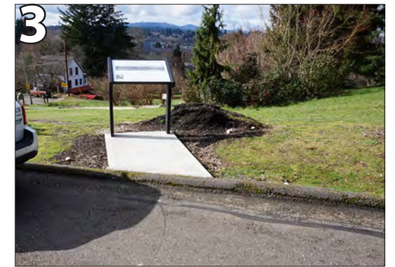
Provide curb ramp to allow for access to signage.
