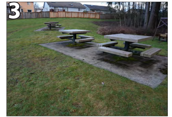
3 Provide ADA accessible pathway to picnic tables.
