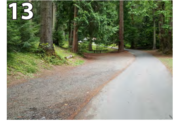
13 No ADA accessible parking. Provide (1) ADA parking space w/ proper signage.
