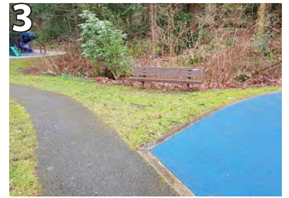
Bench is not accessible. Add accessible route to bench and provide 36" x 48" level pad on one end of the bench.
