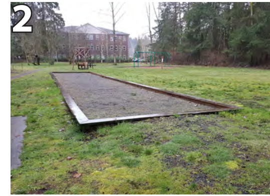
2 Bocce ball court not accessible. Add accessible pathway to court and provide accessible method of entry to allow for access into court.
