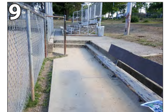
9 Dugout areas inaccessible. Install path or ramp to allow for access.
