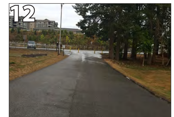
12 Pathway exceeds 1:20 running slope and 1:48 cross slope. Regrade pathway so it is compliant.
