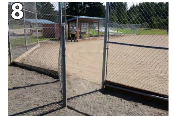
8 Widen fence openings to 36".
