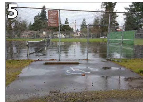
5 Provide ADA accessible parking space for tennis court with proper markings and signage.
