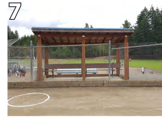
7 Provide 1 space in dugout that can be occupied by a wheelchair.
