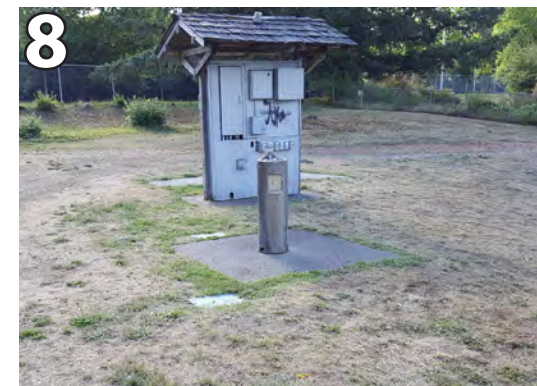
8 Drinking fountain not ADA compliant and not accessible. Replace with ADA complaint drinking fountain and relocate.
