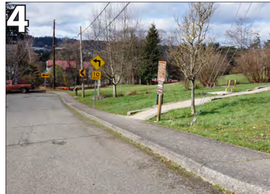
Provide ADA compliant curb ramp to allow access to pathway.
