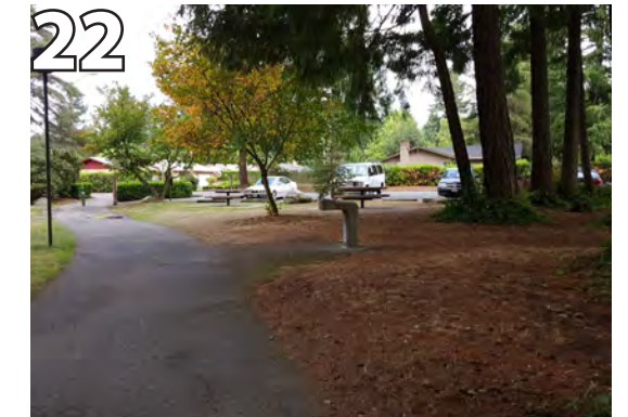
22 Area around drinking fountain too steep. Regrade with a slope no greater than 1:48.
