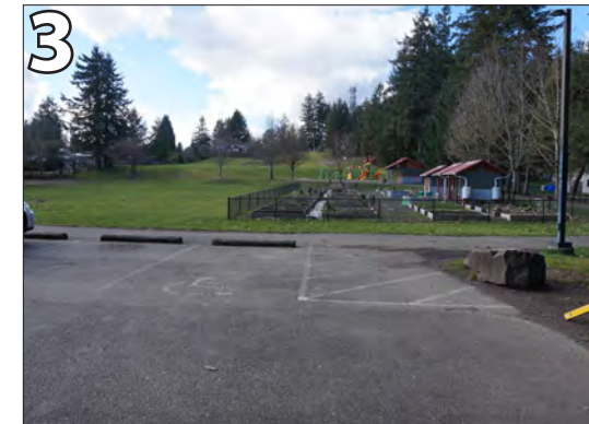
No "Van Accessible" ADA sign.
