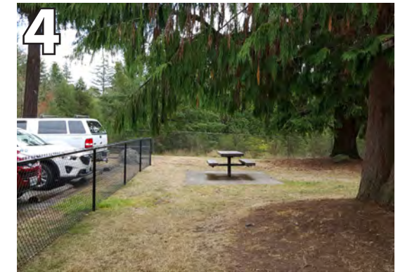
Picnic table not accessible from parking lot and not ADA compliant. Provide ADA compliant pathway and table.
