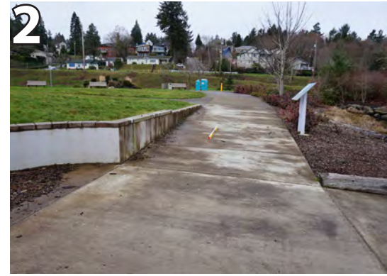
Ramp to boat launch exceeds 5%. Install ADA compliant handrails on either side of ramp.
