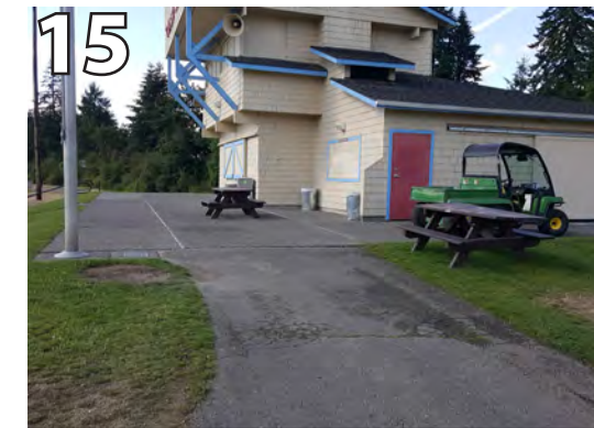
15 Slope exceeds 1:20 and is considered a ramp. Install railings on either side of ramp.
