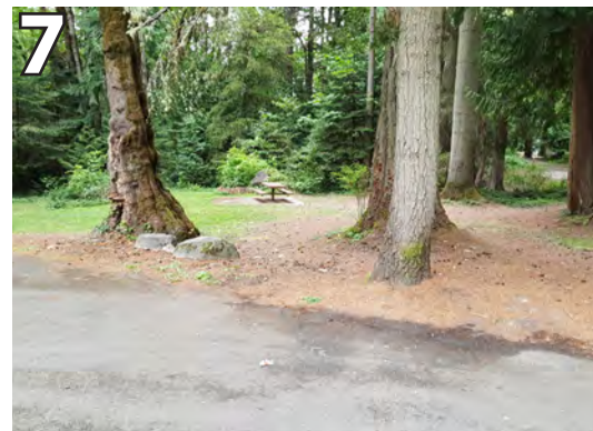
7 No accessible route to picnic table. Provide ADA accessible pathway.
