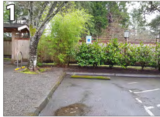
Provide van accessible sign and repaint ADA parking markings so they are clear.
