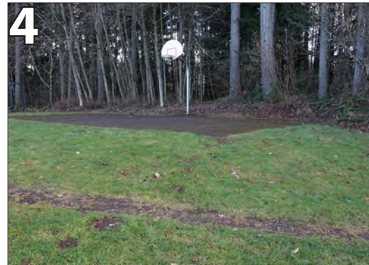
4 Provide ADA accessible pathway to basketball court.
