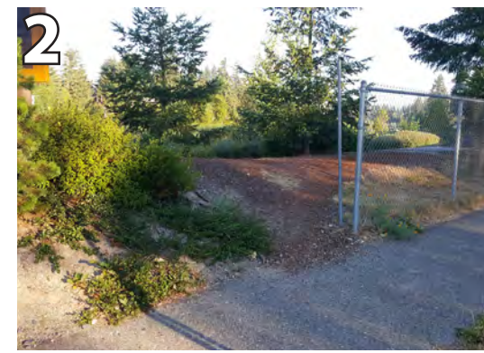
2 No ADA accessible entrance into park from this side of the park. Provide ADA compliant pathway from sidewalk to existing crushed stone pathway.
