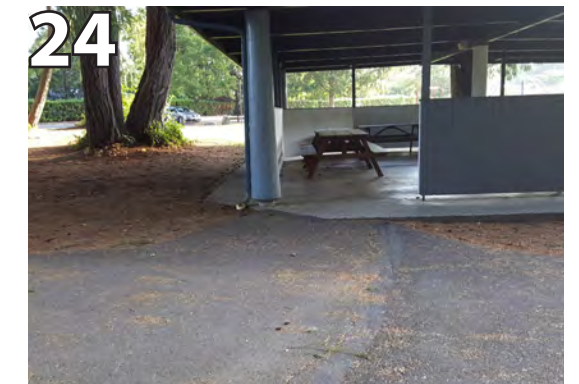
24 Regrade entrance of picnic shelter so that the asphalt and concrete pad are at the same grade.
