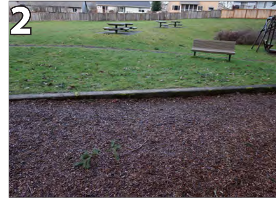
2 Install ADA accessible ramp into EWF area for swing sets.
