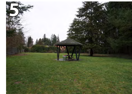
5 No ADA accessible pathway to picnic area. Install 60" wide pathway from existing asphalt to nearest picnic shelter.
