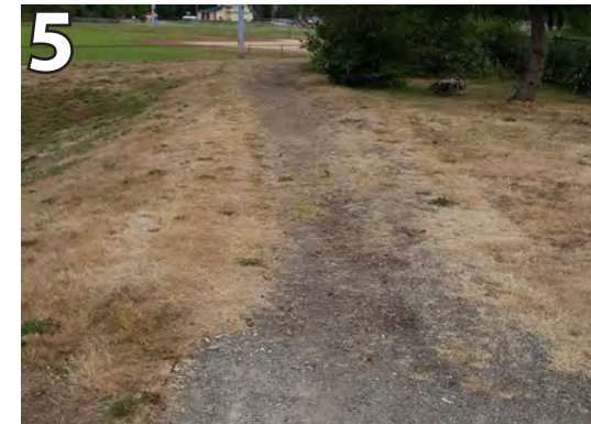
5 Pathway not ADA accessible. Install 60" ADA asphalt pathway.
