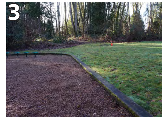
3 Provide ADA curb ramp into play area.
