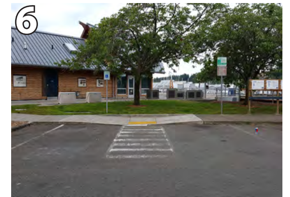
6 Inadequate ADA parking. Provide (3) ADA accessible parking spaces. (1) must be van accessible and have proper curb cuts & signage.
