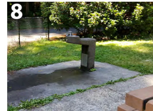
8 Non-compliant drinking fountain.
