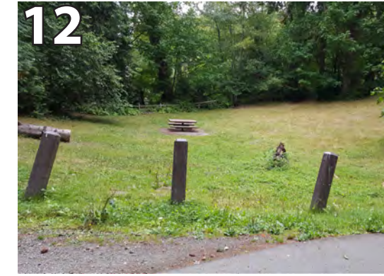
12 Picnic table not ADA accessible. Install ADA accessible pathway.
