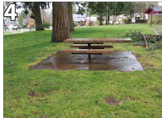
4 Provide ADA accessible pathway to picnic table.
