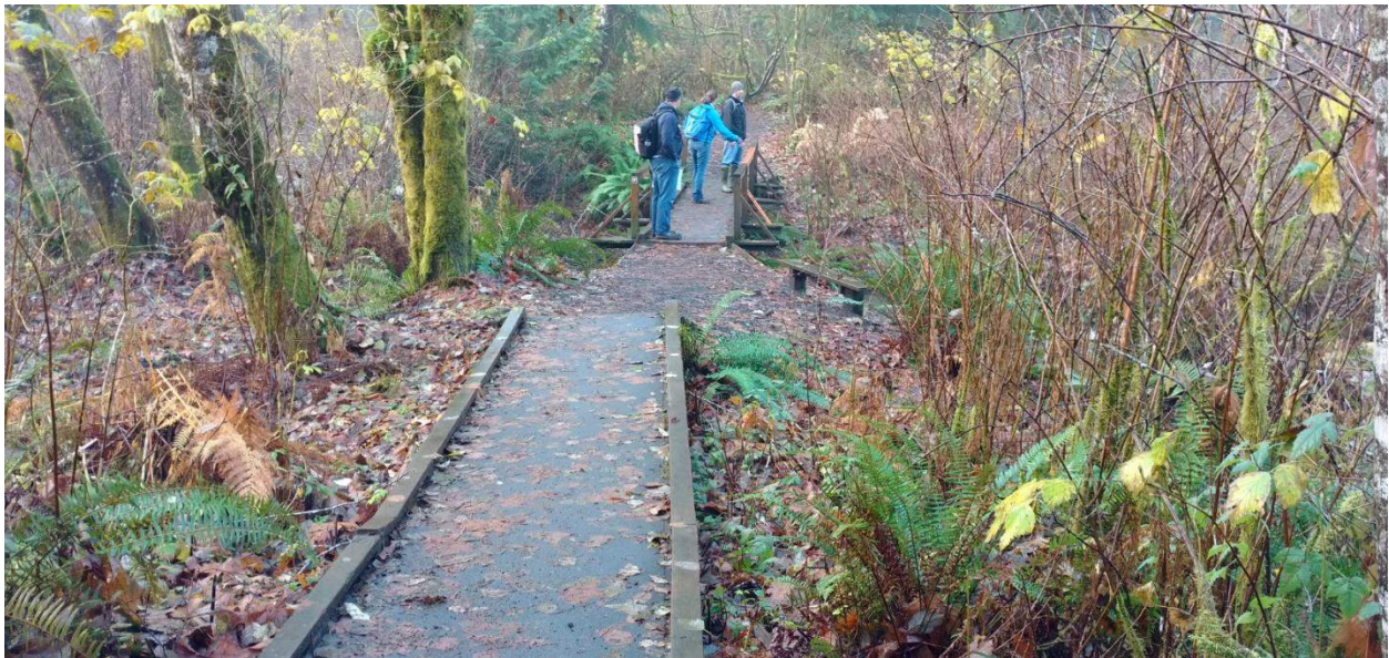
Figure 4. Showing of 4-5-ft wide bridged crossing at Moxlie Creek and associated wetlands.
